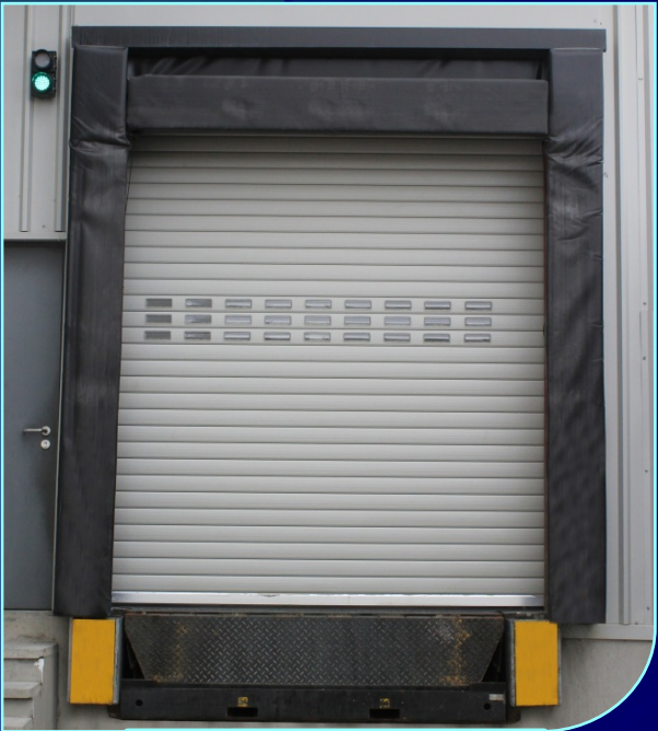
Dock Leveller Installation
